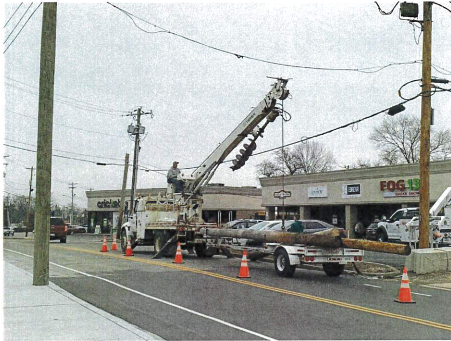
EXISTING POLES BEING REMOVED SO NEW SIDEWALK CAN BE CONSTRUCTED.
