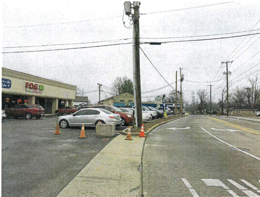
EXISTING POLES TO BE REMOVED SO NEW SIDEWALK CAN BE CONSTRUCTED.
