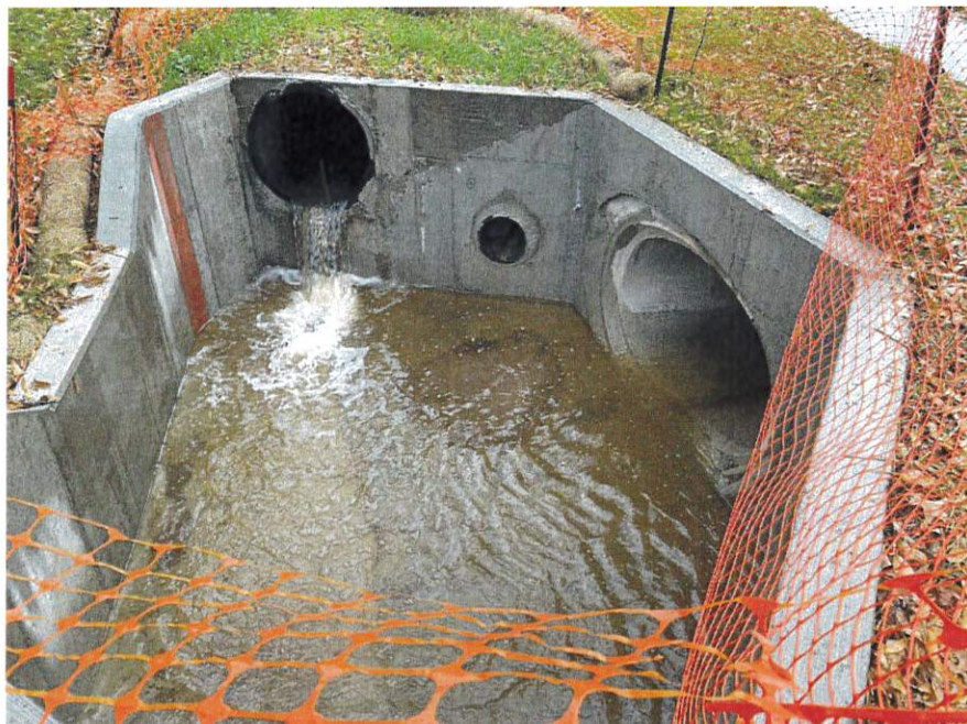
BOX STRUCTURE AT SOUTH CULVERT STILL NEEDS RAILING INSTALLED.
