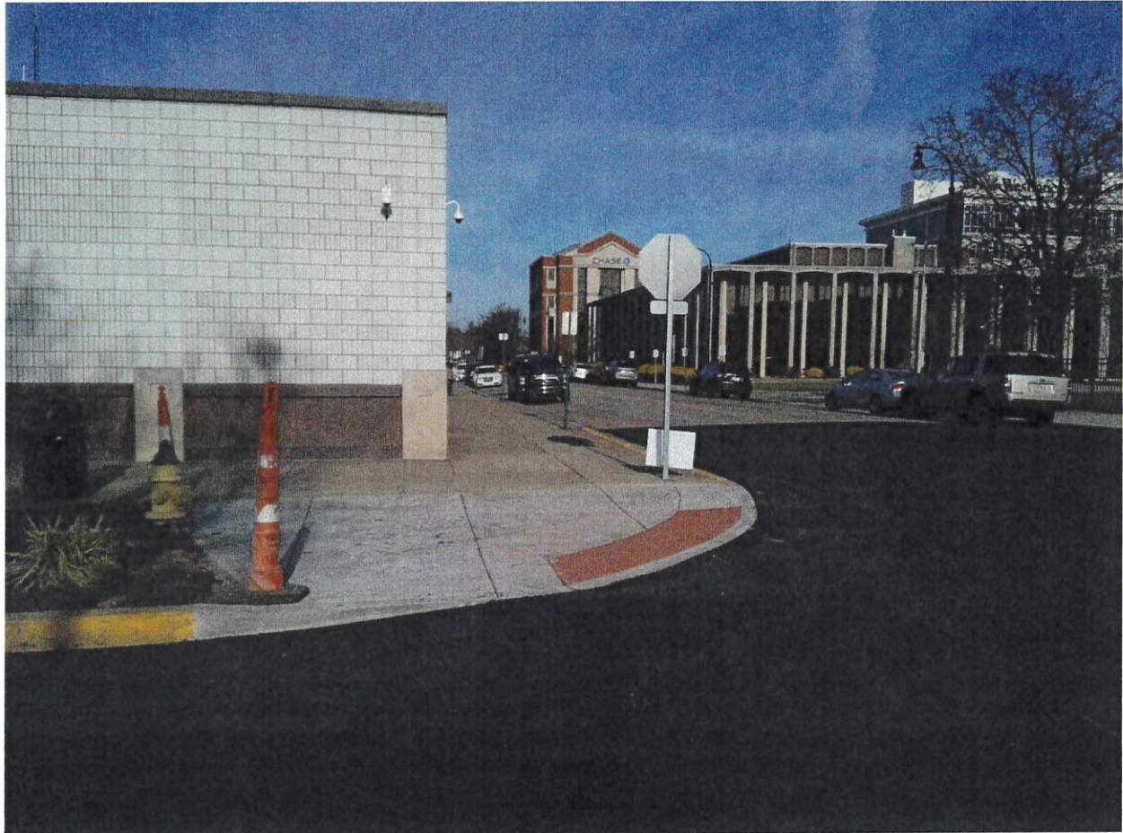
Last curb ramp for the year at Market St. and HMA Surface laid.
