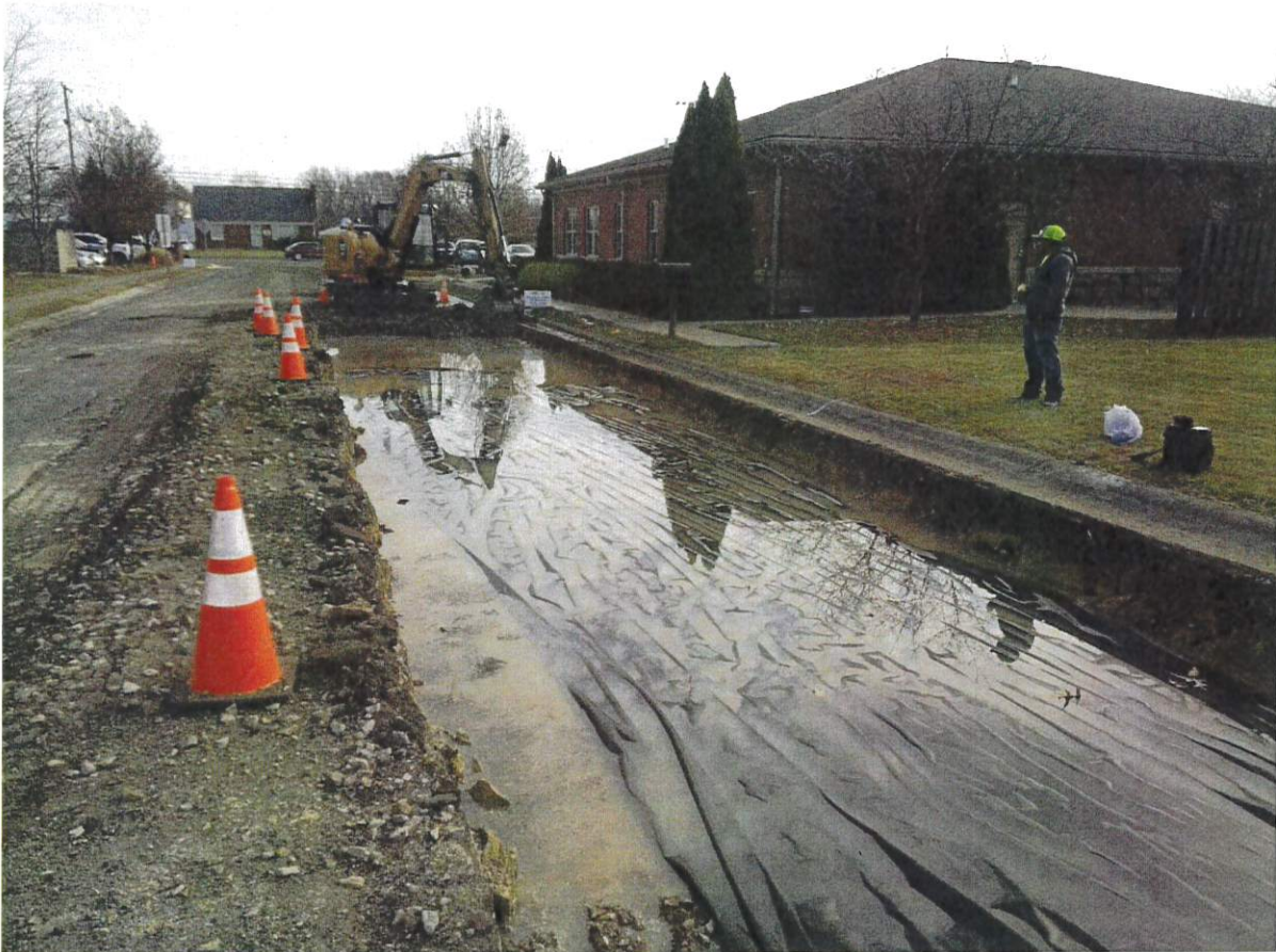
Ellen Court, full depth undercut delayed by water service hit.
