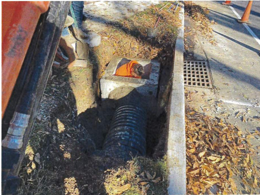
COMPLETING MODIFICATIONS TO TIE-IN STORM LINE ON WEST SIDE OF ROADWAY.
