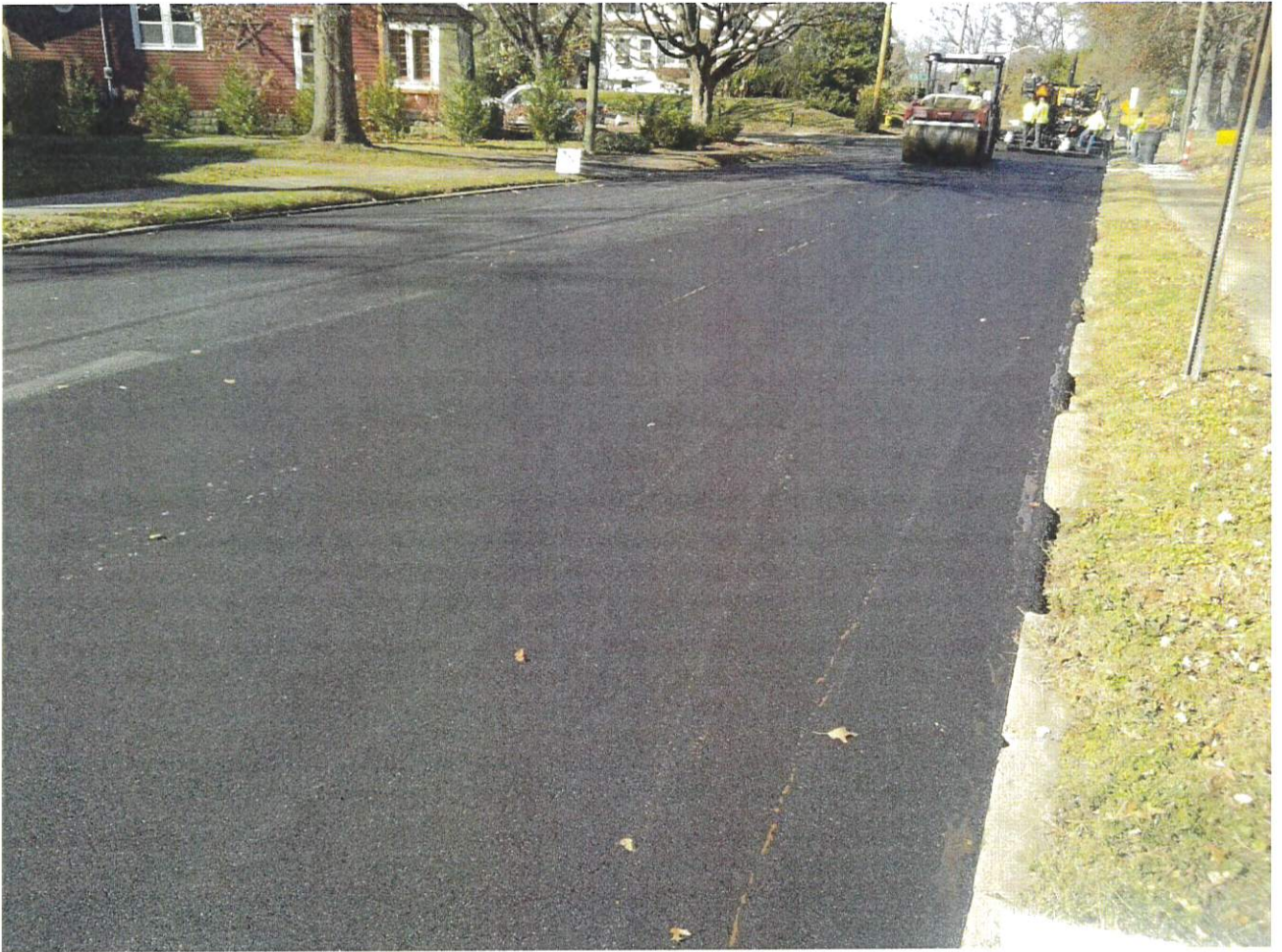
HMA, 9.5mm Surface being laid at Beharrell Avenue.
