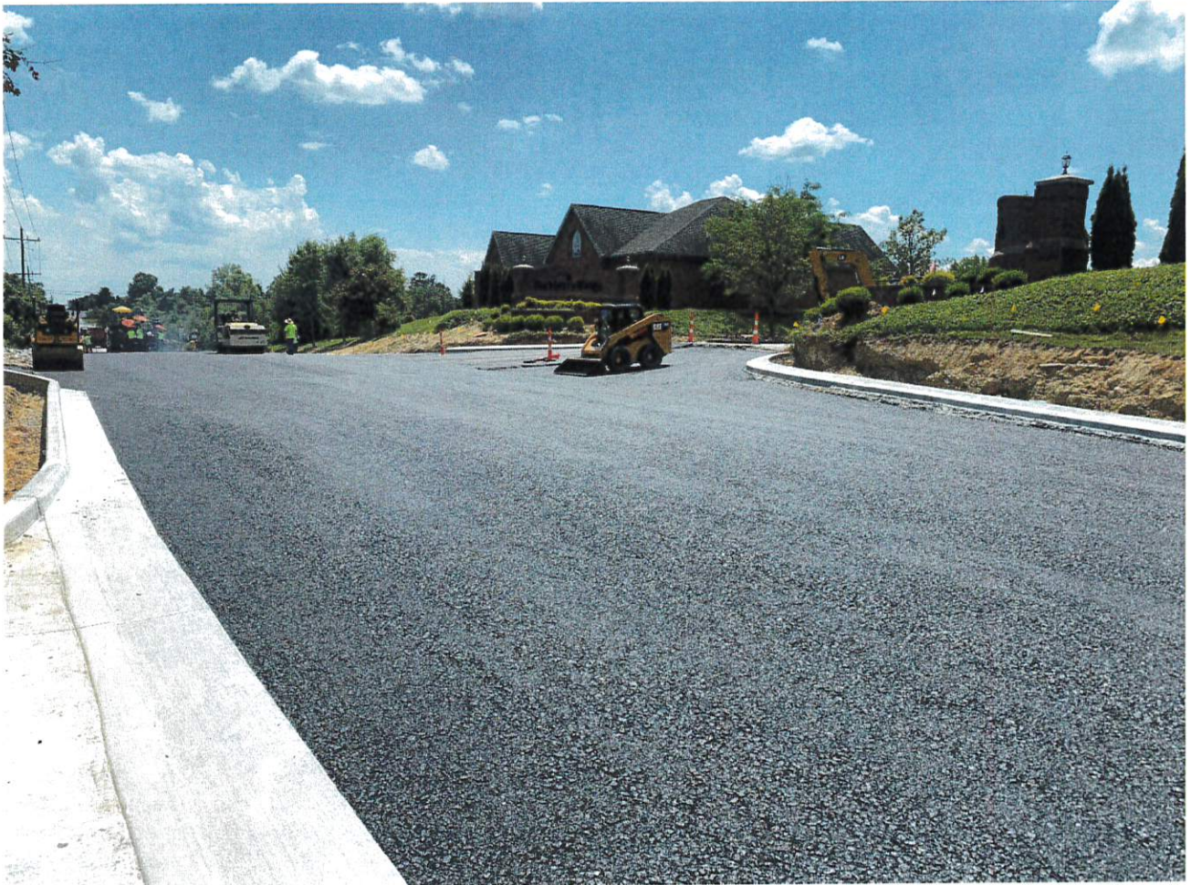
Base layer of HMA installed.
