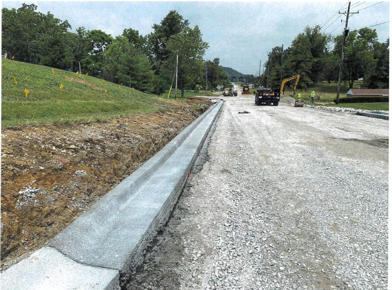
New vertical curb and gutter installed in front of Blackberry Ridge with transition from the new roll curb.
